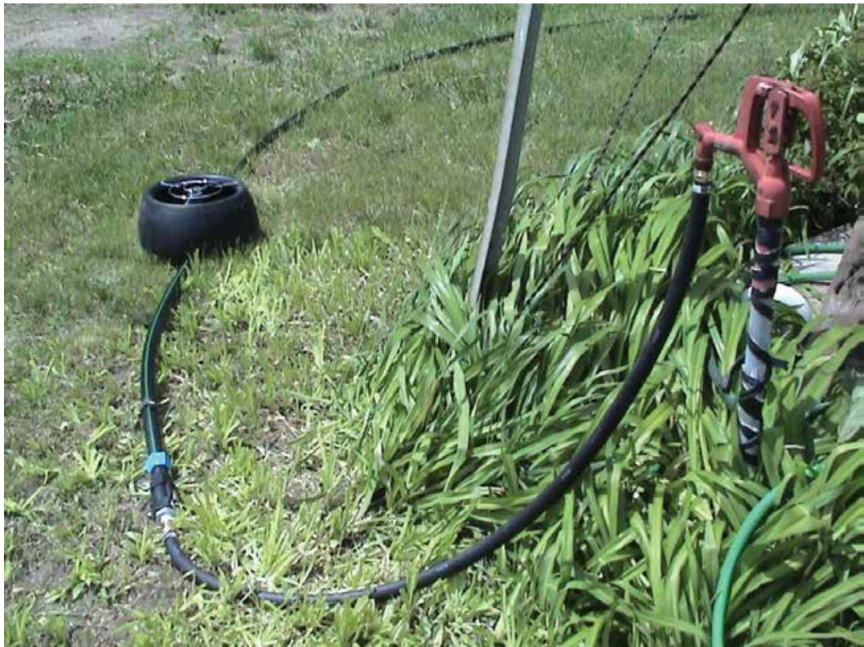
Figure 11. K-Line 1 1/4" tube connected to water hydrant with a Waterman AVP 1 air vent in the pod. Connections made using cam-lock fittings along the length of the tube. Photo credit Jason Gross.
