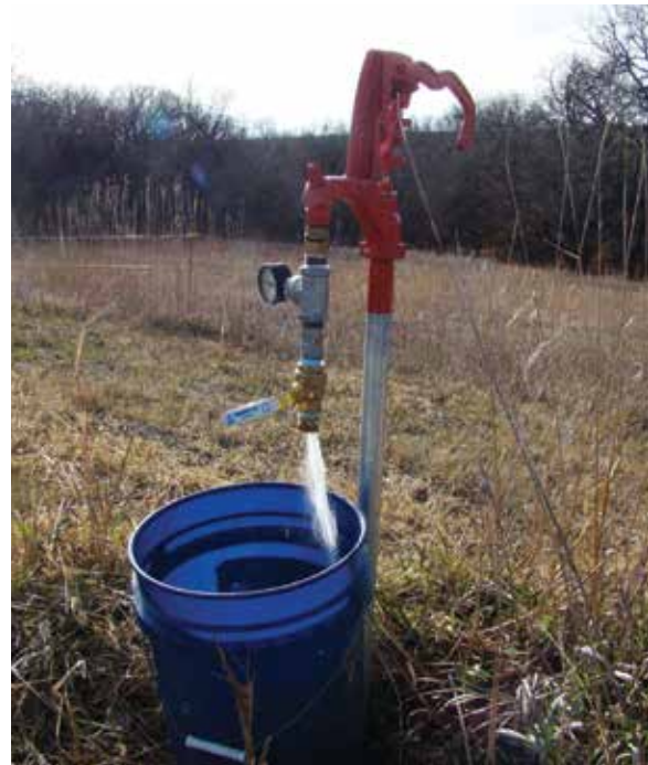
Figure 15. Assembly for measuring water pressure and flow rate from a hydrant. Photo credit Jason Gross.
